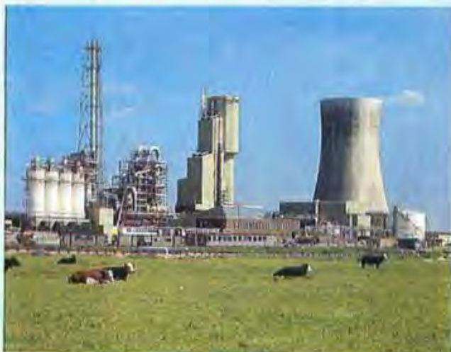
Fig. 10 ICI's 'Pruteen' factory. The tall building in the centre houses the fermentation tanks; on the left are the storage containers; in between is the drying unit.
