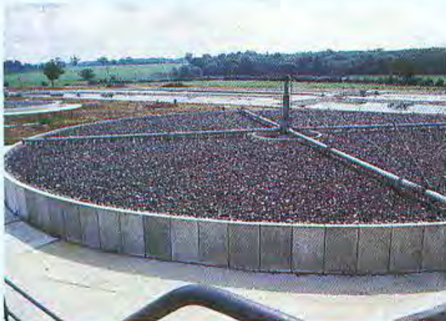
Fig. 5 Sewage treatment. Micro-organisms in the filter beds remove organic matter from the effluent.
